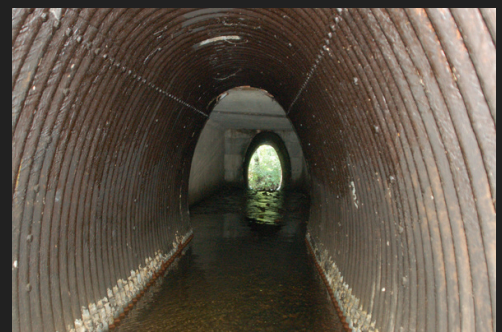
Cow tunnel under Route 46
