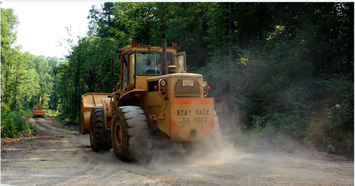
Earth-moving at South Branch Preserve
